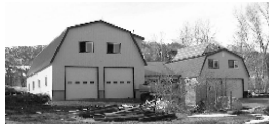
BCRFD Fire Station renovations adding training facility and community center are near completion
